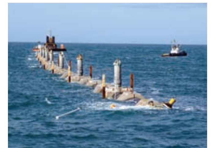
Outfall pipeline during construction.
